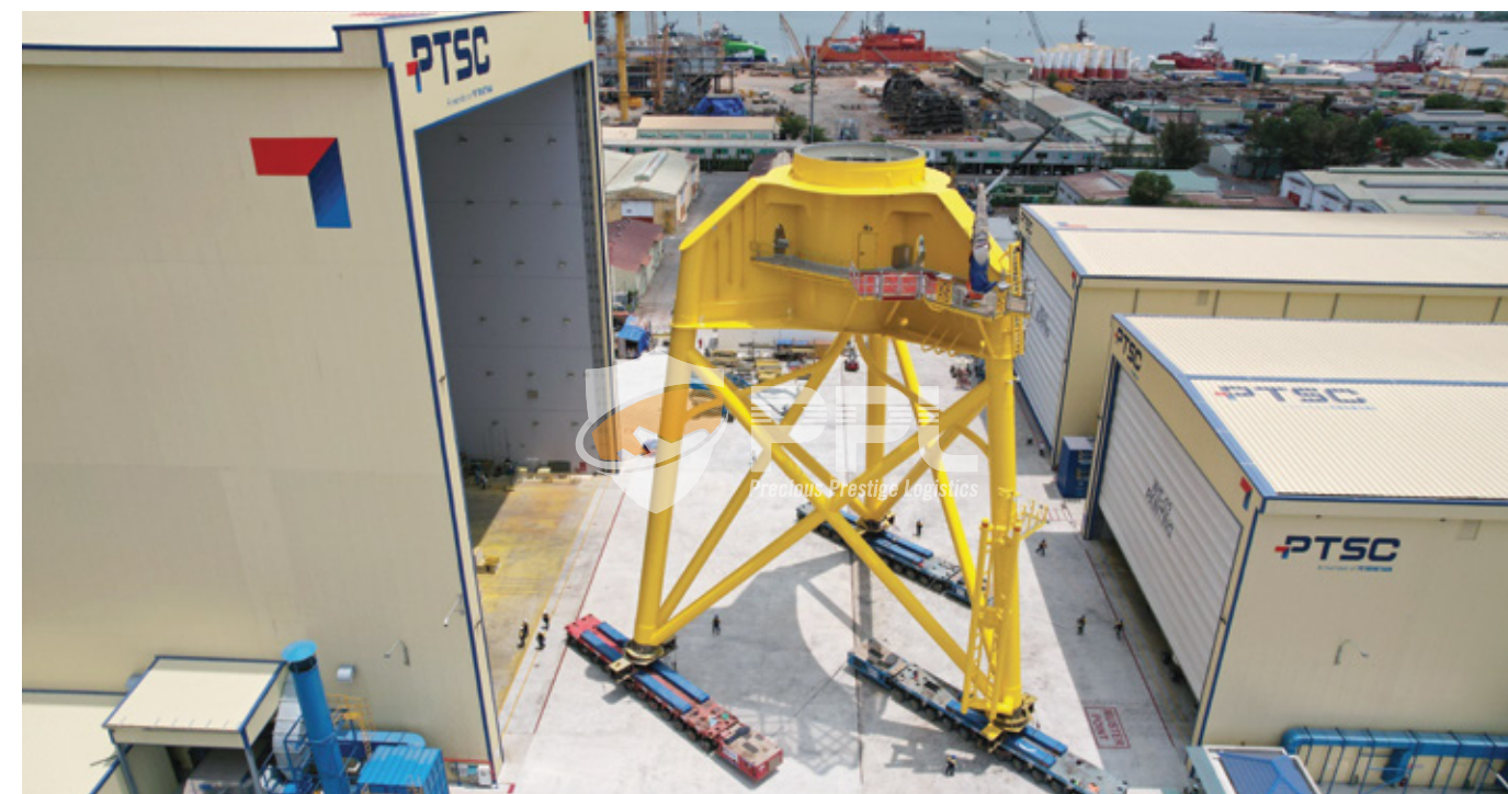
Part 2 (TP+UJ) 24.699 x 31.949 x 35.35 m 770.406 tons
