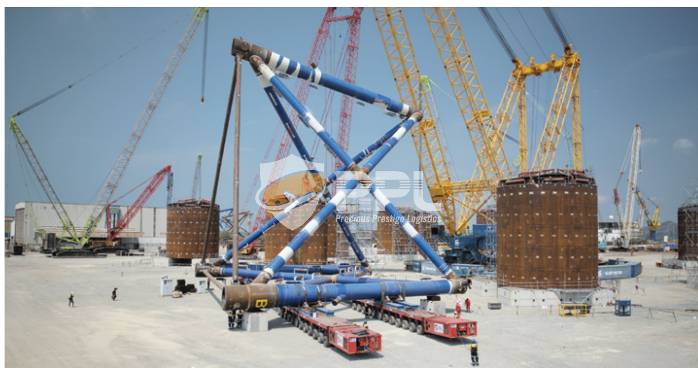
Lower Jacket (LJ) 37.206 x 36.938 x 32.222 m 590.67 tons
