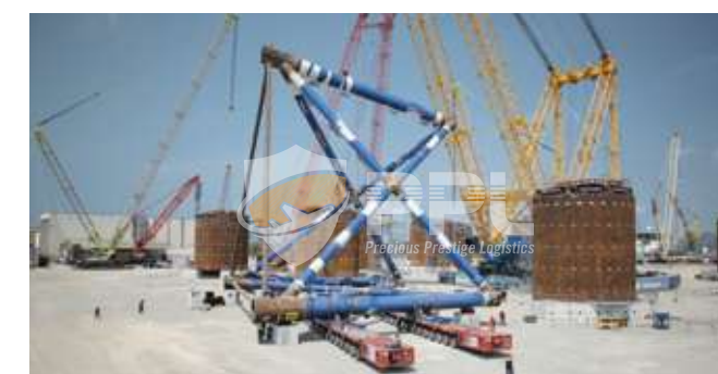
Lower Jacket (LJ) 37.206 x 36.938 x 32.222 m 590.67 tons
