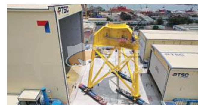
Part 2 (TP+UJ) 24.699 x 31.949 x 35.35 m 770.406 tons
