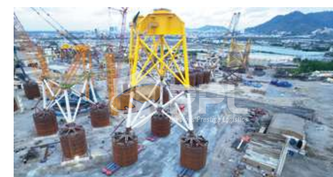
Suction Bucket Jacket 51.596 x 46.566 x 82.040 m 2,387 tons
