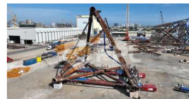
Upper Jacket (UJ) 27 x 24 x 24 m 325.7 tons
