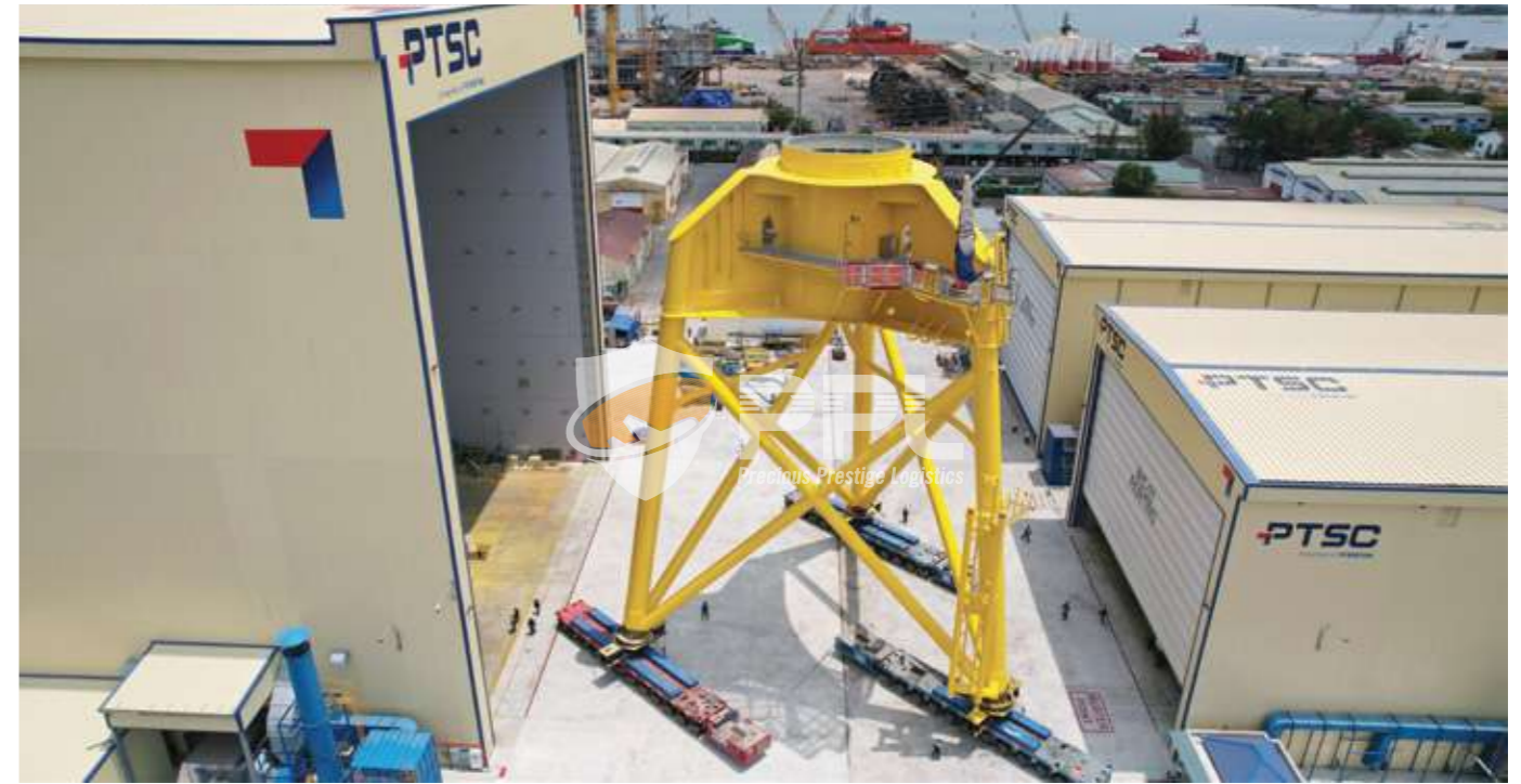
Part 2 (TP+UJ) 24.699 x 31.949 x 35.35 m 770.406 tons
