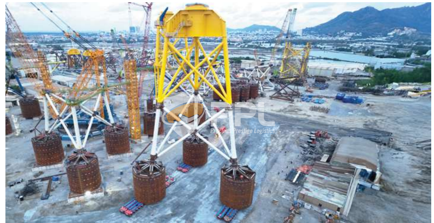
Suction Bucket Jacket 51.596 x 46.566 x 82.040 m 2,387 tons
