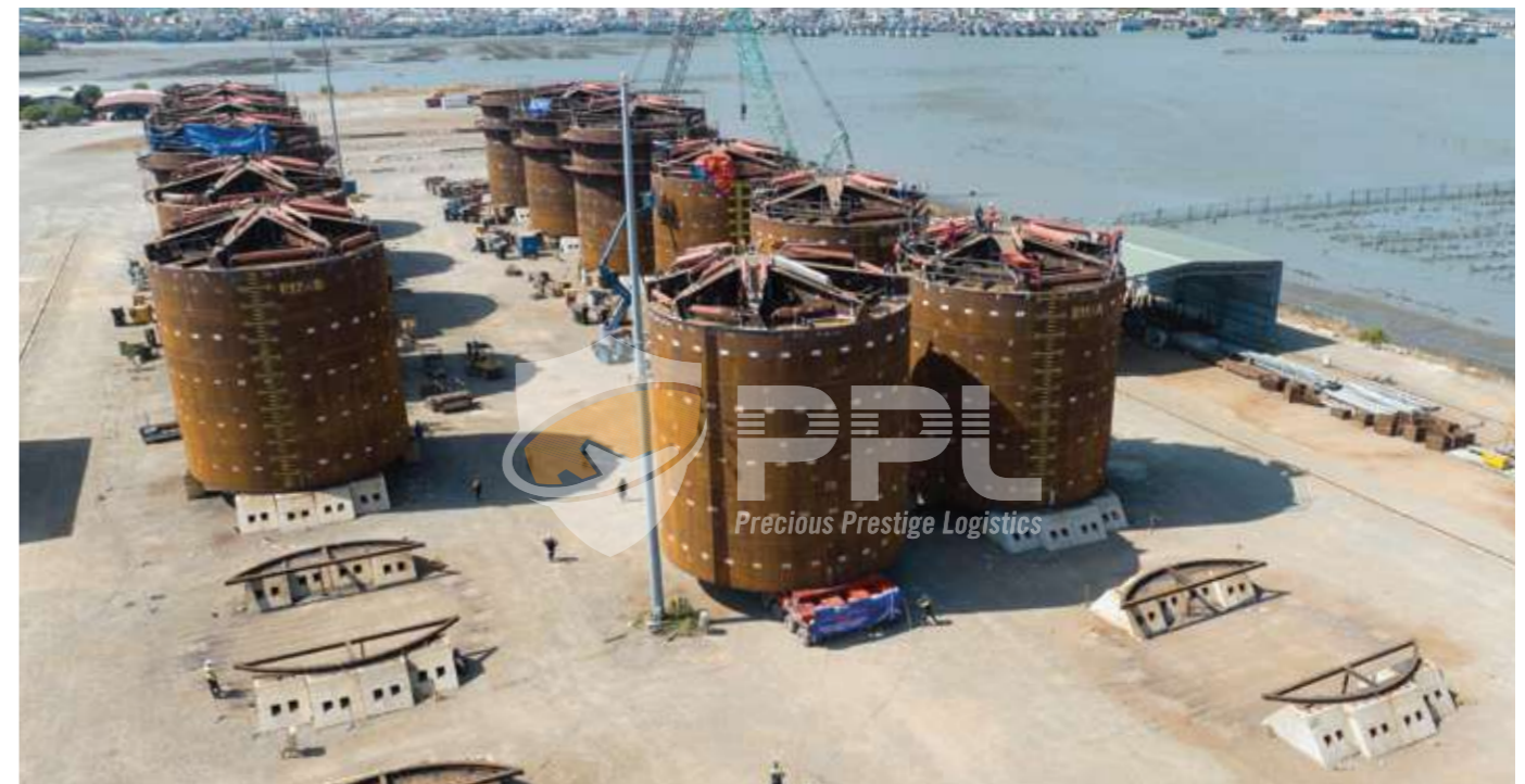
Suction Bucket (SB) Ø13-14 x 16.774 m 350.915 tons
