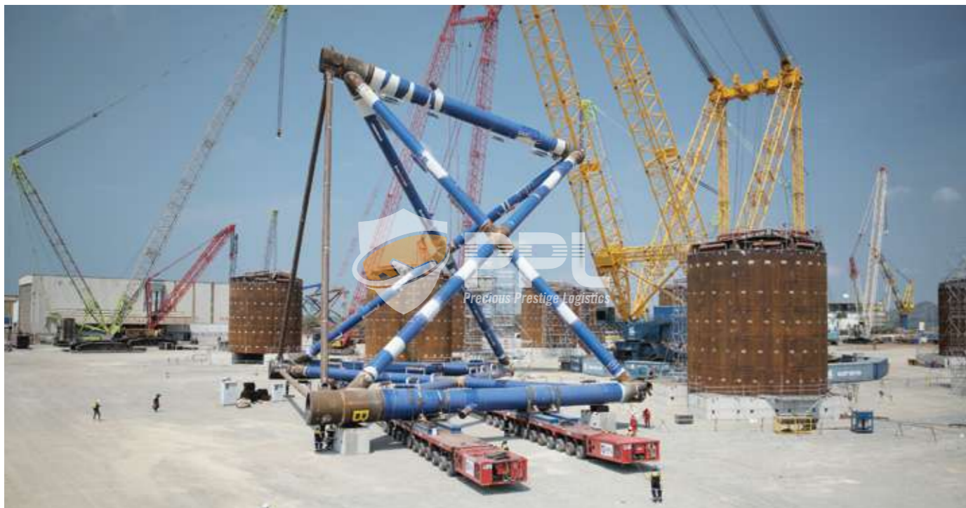
Lower Jacket (LJ) 37.206 x 36.938 x 32.222 m 590.67 tons
