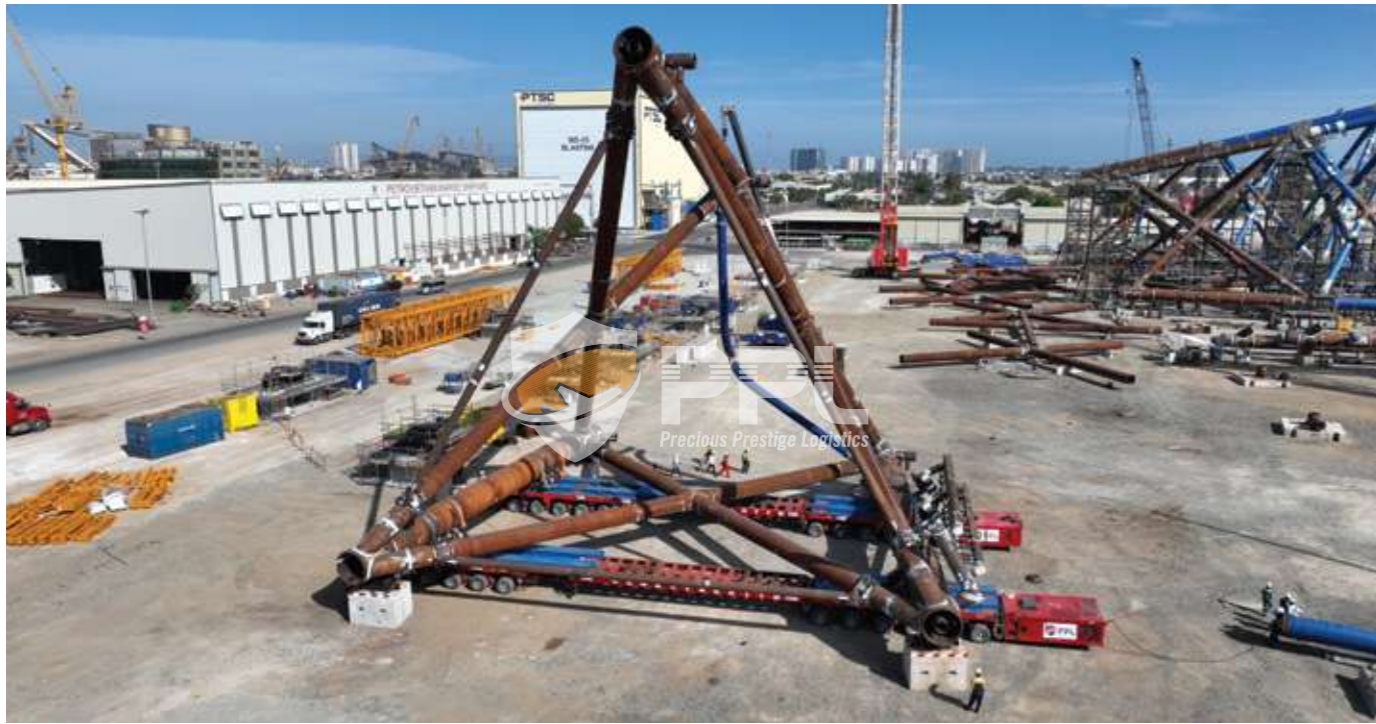
Upper Jacket (UJ) 27 x 24 x 24 m 325.7 tons
